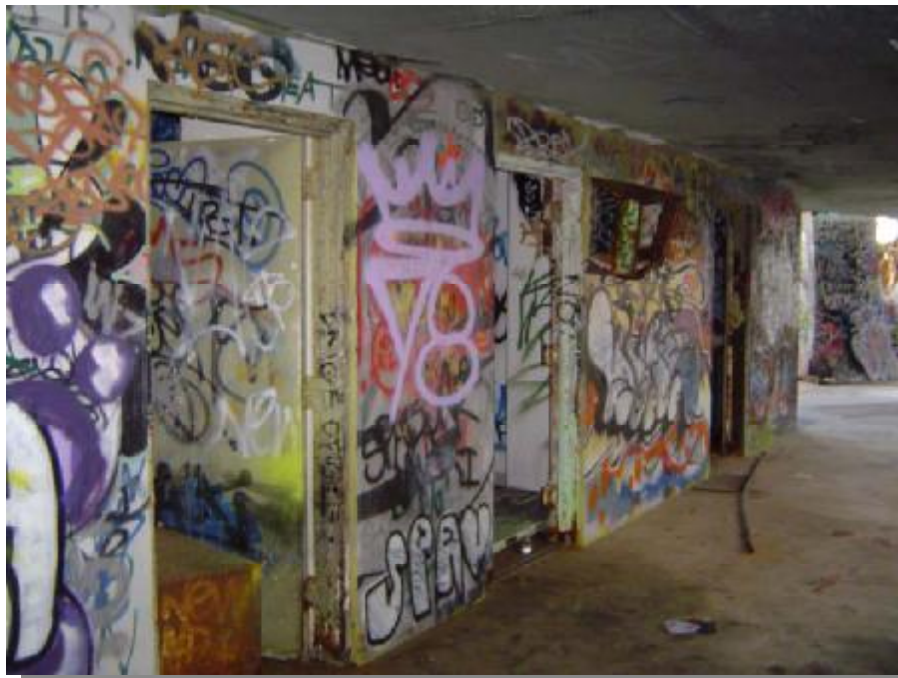
20- Typical Building Condition
