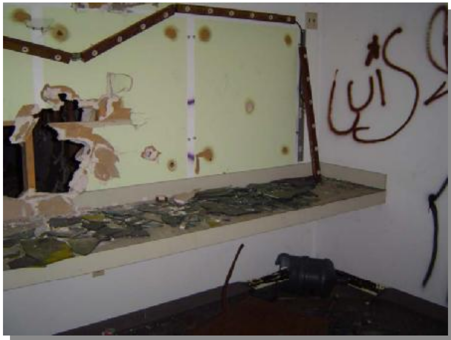
26- Dressing Room Area General Building Condition
