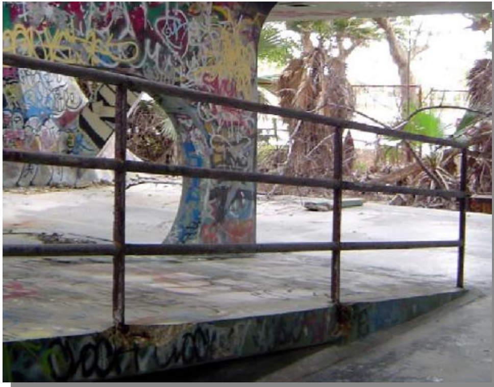
12- Railing and Imbed Condition
