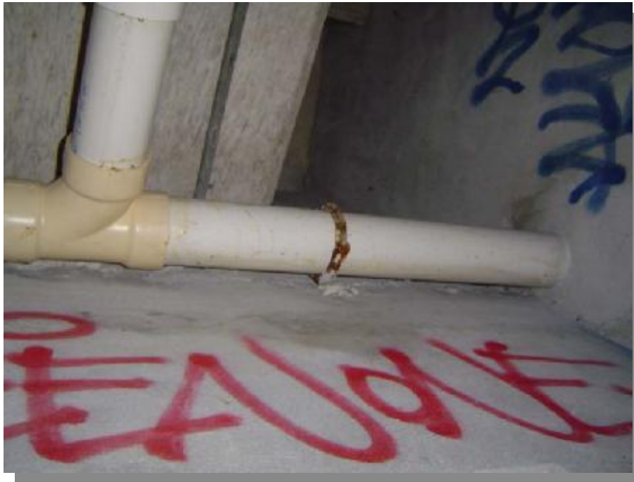
47- PVC Sanitary Pipe Retro Fit
