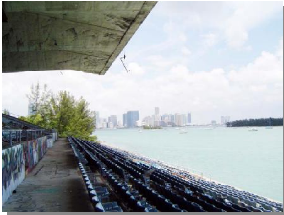
56- Lighting Fixture Hanging by Wire
