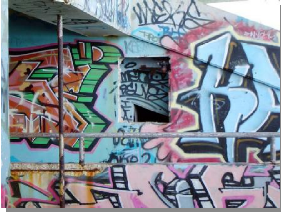
66- Main Ramp Support Beam Deterioration
