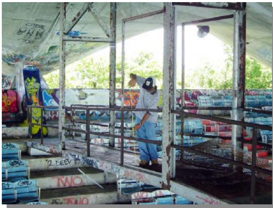
32- Access to Control Booth
