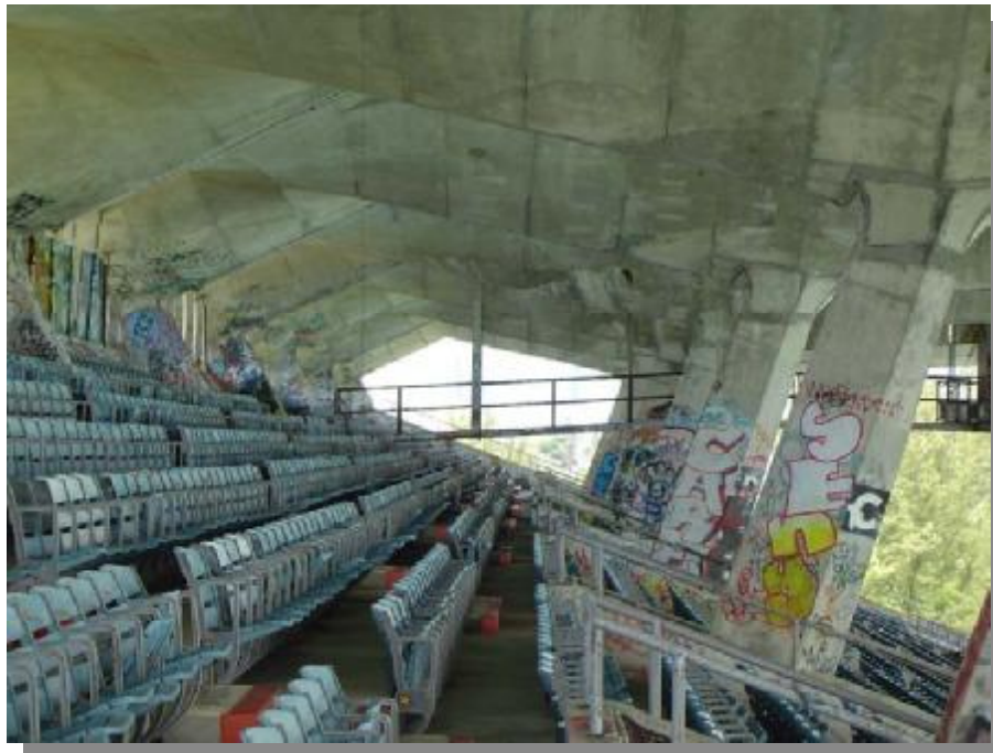
30- Typical Condition Grand Stand Seating Area
