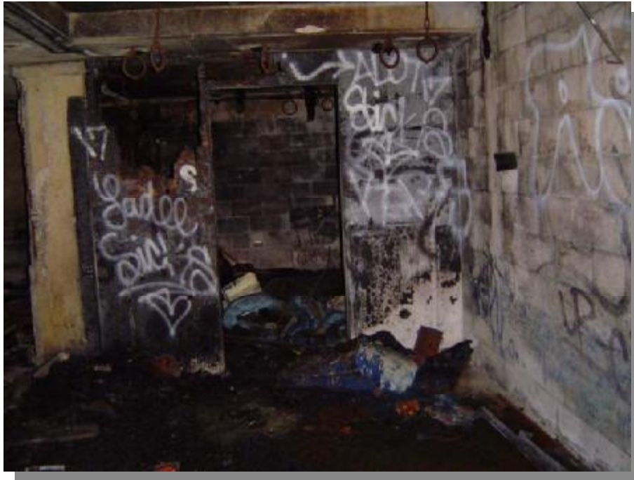
17- Typical Building Condition
