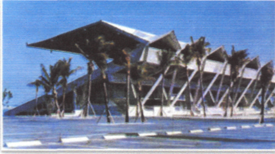
The 6,500-seat grandstand stadium, currently unoccupied, is built entirely of poured concrete and features a dramatic cantilevered fold-plate roof.
