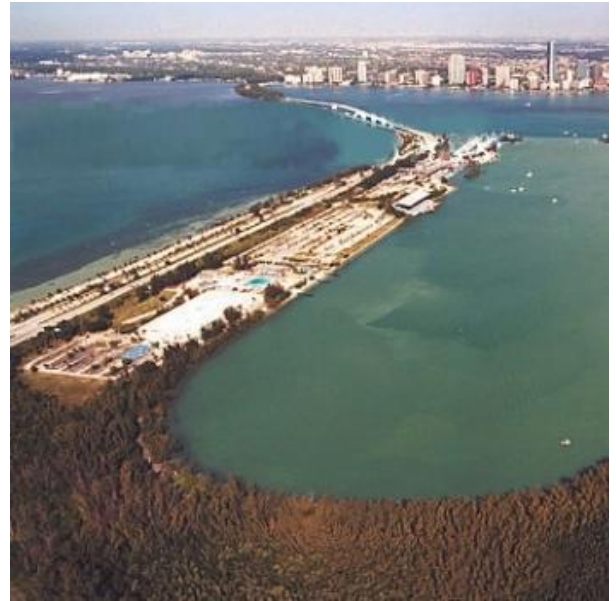
Miami Marine Stadium and basin
