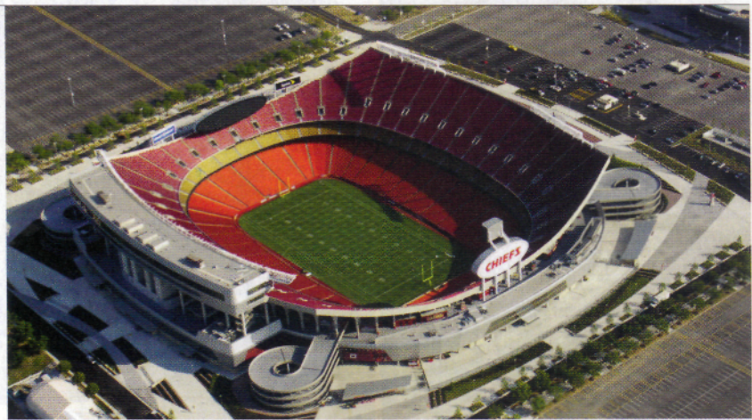
Arrowhead Stadium, in Kansas City, Missouri, recently underwent a substantial modernization that enhanced the 38-year-old structure's amenities without diminishing its traditional feel.
